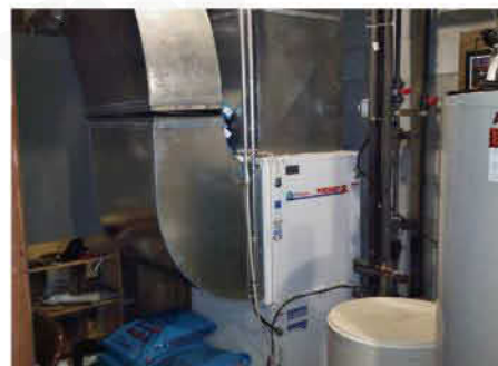
Midkiff's geothermal system produces 70° Fahrenheit (21° Celsius) air from well water at a temperature of 50° F (10° C).
