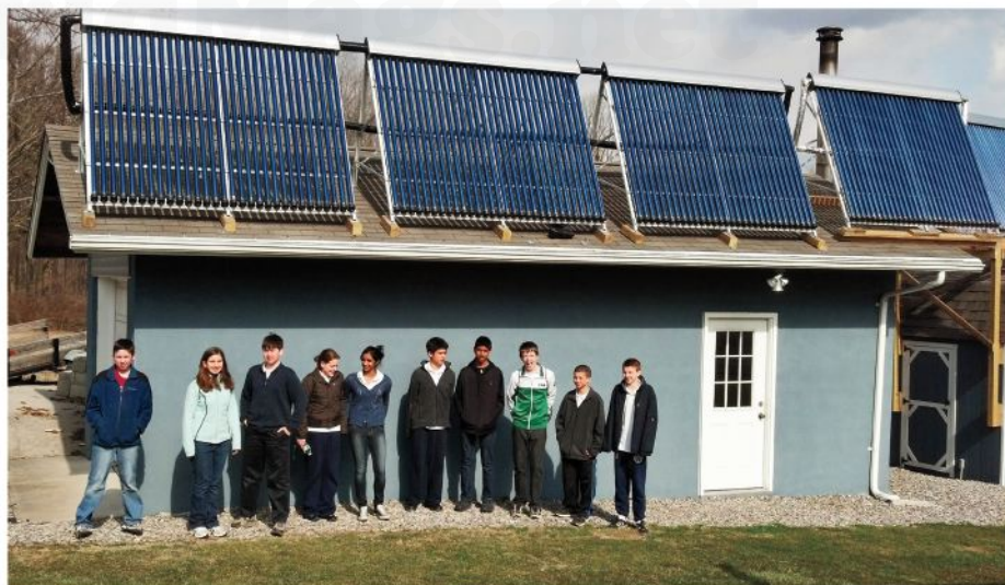
The newest energy-saving addition is this hybrid solar hot-water system. On sunny days, it can heat both houses on the property. Here, a visiting school group poses underneath it.
