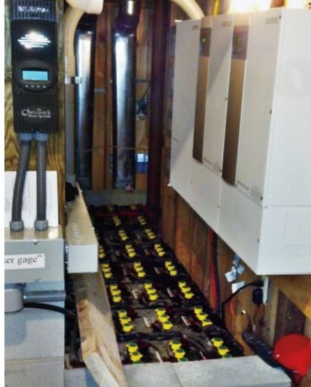
This photo shows the inverters (that convert the direct current that the photovoltaic array produces to more usable alternating current) and the battery bank that stores power for evening or cloudy-day use.
